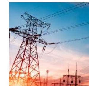
LOW VOLTAGE TEST
